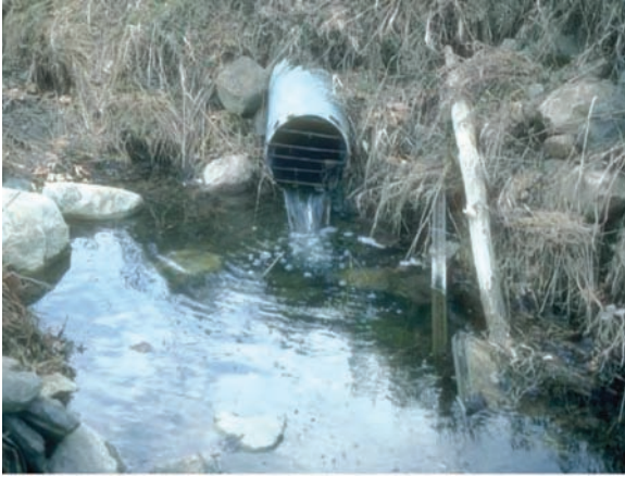
Figure 17.19. Subsurface drain line discharges into an edge-of-field ditch, diverting groundwater to surface waters.
